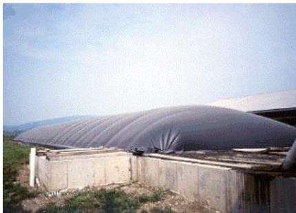
Methane collected inside air-tight plastic cover
